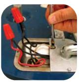
Consult the Installation Instructions and the wiring diagram and labels on the water heater. Make sure your home's wiring and circuit breakers are in good condition and are correct for the model you are installing. Connect the power wires and the green or copper ground wire. The ground wire must be connected to the water heater's green ground screw.
