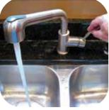
Open a nearby hot water faucet. At first, you'll just get air from the faucet. then sputtering, and finally, on, the upper element will a full flow. Then, let the "hot" water run full for three minutes to ensure the tank is completely full. The tank must be completely full of water before connecting electric power or you will burn out (dry fire) the upper heating element.
