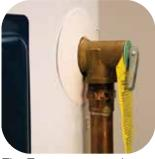
The Temperature and Pressure Relief Valve (T&P) is an important safety device. It opens to relieve pressure if the water temperature or pres- of no more than 6 inches sure is too high. Use the new T&P that came with your new water heater. Don't reuse the old T&P valve.
