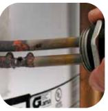
If you have no hot water (not even warm) after a few hours, check to make sure the water heater is getting power. If you have power but no hot water, the upper element may have been "dry fired" and will need to be replaced. Replacement elements are inexpensive and widely available.
