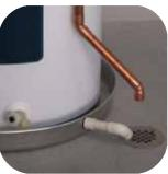
The Temperature and Pressure Relief Valve (T&P) discharge pipe should be terminated near a floor drain with an air gap between the end of the discharge pipe and the drain. Some localities require terminating the T&P discharge pipe outside. In cold climates, we recommend using a floor drain. In all cases, follow the codes for your location. Warning: Do not plug or cap the T&P discharge pipe.
