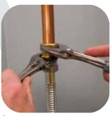
Check the water connections for leaks. Most leaks are due to problems with the inlet or outlet water connections (not a tank leak).
