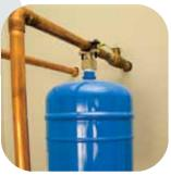
Almost all homes have check valves in the plumbing system and now need a thermal expansion tank installed near the water heater. The expansion tank is attached to the cold water inlet line. To operate properly, the expansion tank must be pressurized with air. Refer to the expansion tank's instructions for details.
