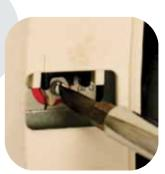
The upper and lower thermostats are both set at the recommended temperature setting of 120° Fahrenheit at the factory. Higher temperatures increase the risk of scalding. See the Installation Instructions and the water heater's labels for detailed instructions and important safety information about scalding.
