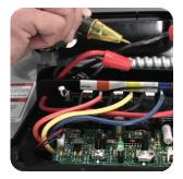
Because circuit breakers can be mismarked, also check the circuit with a circuit tester or meter before performing any work.
