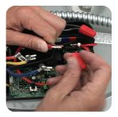
Insert the black and red power wires into the Field Wiring Compartment. *Connect the power wires using wire nuts.*
