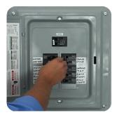
*Now turn electric power back ON.* The Control Board will perform a diagnostic check that takes about 10 minutes. It will take about 2 hours for the tank of cold water to heat up.
