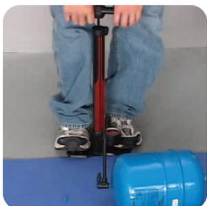
Adjust the air pressure to equal the maximum water pressure in the home. Use a hand pump - **NOT** an air compressor - or you may rupture the bladder.
