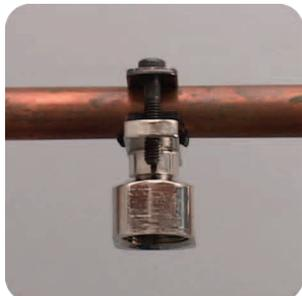
Follow the installation instructions that came with your Thermal Expansion Tank. Connect the tank to the cold water line. Solder a T-Fitting *or use a Saddle Valve that bolts on, no soldering needed.*
