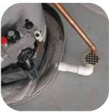
The Temperature and Pressure Relief Valve (T&P) discharge pipe should be terminated near a floor drain with an air gap of no more than 6 inches between the end of the discharge pipe and the drain. Some localities require terminating the T&P discharge pipe outside. In cold climates, we recommend using a floor drain. In all cases, follow the codes for your location. Warning: Do not plug or cap the T&P discharge pipe.
