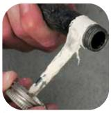
Install the gas pipe using pipe joint compound (or Teflon® tape) approved for fuel gas on all threaded connections. Keep the pipe joint compound from getting inside the gas line or gas control valve. If you are using a flexible gas line connector, follow the instructions that came with the flexible connector (most don't need pipe joint compound). Reconnect the gas line union.
