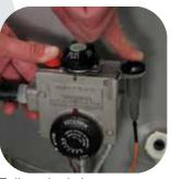
Follow the lighting instructions on the water heater's label. Because the water heater is new and there is air in the gas line, it may take several attempts to light the pilot.
