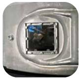
Your new water heater is more energy efficient than older models and has a smaller pilot light which can sometimes be hard to see. You may have to darken the room and look carefully through the sight tion about scalding. glass in order to see the pilot light.
