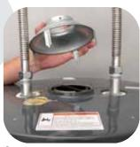
Connect the vent pipe to the water heater's draft hood. Use sheet metal screws. Don't reuse the old draft hood—always use the new draft hood supplied with your new water heater. See the Installation Instructions for important safety information about venting and construction details.
