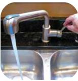
Open a nearby hot water faucet. At first, you'll just get air from the faucet, then sputtering, and finally, up. You may hear drips a full flow. Then, let the "hot" water run full stream droplets hit the burner) or for three minutes to ensure the tank is completely puddle. Condensation is full. The tank must be completely full before light- Condensation should go ing the pilot.
