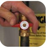
Turn the main gas supply valve OFF. Also, turn the gas control knob on the old water heater off. Open a hot water faucet and let the hot water run until cool. Allow the old water heater and vent pipe to cool.
