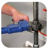
Disconnect the gas line at the union (you'll need two wrenches for that). Remove the gas pipe from the old water heater—you may be able to reuse it. Save the union, too. Next, remove the water lines and the old water heater. Install the new water heater (in a metal drain pan).
