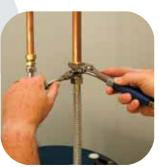
Install the hot and cold water lines. The water heater inlet and outlet connections contain non-metallic parts. Don't solder pipe directly to these connections. Instead, solder threaded adapters to short pieces of pipe so that soldering is done a foot or so from the water heater connections. Open the cold water supply valve and fill the tank.
