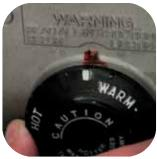
Adjust the temperature to 120°F. Higher temperatures increase the risk of scalding. See the Installation Instructions and the water heater's labels for important safety informa-
