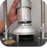
Disconnect the vent pipe from the draft hood. Inspect the old vent pipes for corrosion, obstructions, leaks or other damage, and repair or replace if necessary. Gas water heaters must have free access to adequate combustion air and must be properly vented. The Installation Instructions explain these requirements, and they must be followed for safe operation.
