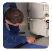
Vacuum any remaining lint from the bottom of the water heater using the vacuum cleaner's crevice tool.
