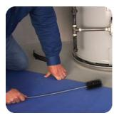
If the water heater is in a drain pan, use a brush with a flexible handle using an in and out motion and vacuum the brush. Repeat brushing and vacuuming until the brush is completely clean.
