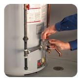
After cleaning the FVIR Flame Arrestor and Filter Screen, try relighting the pilot using the instructions on the water heater's label. If the pilot still won't light, a service technician may be needed to perform a more thorough cleaning or to check for other problems.
