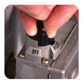
To clean the FVIR system, first turn the water heater off. **Allow the burner to cool for about 15 minutes**.
