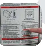
Follow the lighting instructions on the water heater's Instructions have a handy Check List. Review each Instructions Manual and on corrections or repairs as necessary. It's important that every step has been successfully completed before attempting to light the water heater. With the gas valve on/off switch in the OFF position, plug the water heater into a standard wall outlet that is properly grounded.
