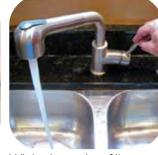
While the tank is filling, it is important to open a hot water faucet and let the water run full for at least three minutes to ensure all the air is out and the tank is completely full of water. Check all connections for water leaks. Almost all leaks are at connections, not a tank leak.
