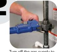
Turn off the gas supply to the water heater at the manual shut-off valve. Turn gas control knob to the OFF position. Disconnect the gas line at the union (you'll need two wrenches for that). Remove the gas pipe from the old water heater—you may be able to reuse it. Save the union, too.
