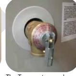
The Temperature and Pressure Relief Valve (T&P) is an important or pressure if the water that came with your new water heater. Don't reuse the old T&P valve.
