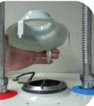
Connect the vent pipe to the water heater's unique draft hood (note that the flat sides of the draft hood face water pipes.) Use sheet metal screws. Don't reuse the old draft hood—always use the new draft hood supplied with your new water heater. See the Installation Instructions for important safety information about venting and construction details.
