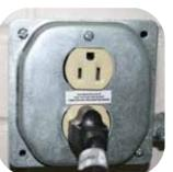
This high-efficiency gas water heater requires a 120VAC, 60 Hz electrical supply. A 10-foot cord with three-pronged plug is supplied (no extension cords are permitted) and the outlet must be properly grounded. Follow local codes. See Installation Instructions for details.
