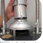
Be certain that the vent has cooled before handling. Disconnect the vent pipe from the draft hood. Inspect the old vent piping for corrosion, obstructions, leaks, or other damage, and repair or replace if necessary. Gas water heaters must have free access to adequate combustion air and must be properly vented. The Installation Instructions explain these requirements, and they must be followed for safe operation.
