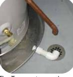
The Temperature and Pressure Relief Valve (T&P) discharge pipe should be terminated near a floor drain with an air gap of no more than 6 the drain. Some localities require terminating the T&P discharge pipe outside. In cold climates, we recommend using a floor drain. In all cases, follow local codes. Read the Instruction Manual for important details. Warning: Do not plug or cap the T&P discharge pipe.
