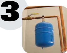
Almost all homes have check valves in the plumbing system and homes now need a thermal expan- safety device. It opens sion tank installed near the to relieve temperature water heater. The expansion tank is attached to the cold water inlet line. To operate properly, the expansion tank must be pressurized with air. Refer to the expansion tank's instructions for details.
