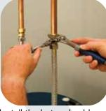
Install the hot and cold water lines. If using quick connect fittings, pipe compound or Teflon® tape is not required. If using flexible or solid connections, the threaded fittings would require pipe compound approved for potable water or Teflon® tape on the threaded fittings. Turn the cold water supply back on and check for leaks. Do not solder pipes while they are connected to the water heater. Use thread-
