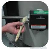
Turn the gas supply valve ON. Brush soap solution on all gas line connections label. The Installation and look for bubbles. Use plenty of soap solution. Gas is under low pressure, item in the Installation and it may take some time for bubbles to appear. the Check List and make If you see any bubbles, correct the leak and retest. DO NOT check with
