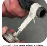
Install the gas pipe using pipe joint compound (or Teflon® tape) approved for fuel gas on all threaded connections. Keep the pipe joint compound from getting inside the gas line or gas control valve. If you are using a flexible gas line connector, follow the instructions that came with the flexible connector an open flame. (most don't need pipe joint compound). Reconnect the gas line union.
