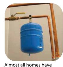
check valves in the plumbing system and homes now need a thermal expansion tank installed near the water heater. The expansion tank is attached to the cold water inlet line. To operate properly, the expansion tank must be pressurized with air. Refer to the expansion tank's instructions for details.
