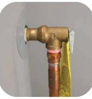
The Temperature and Pressure Relief Valve (T&P) is an important safety device. It opens to relieve temperature or pressure if the water temperature or pressure is too high. Use the new T&P that came with your new water heater. Don't reuse the old T&P valve.
