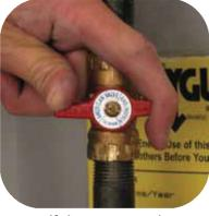
Turn off the gas supply to the water heater at the manual shut off valve. Turn gas control knob to the OFF position. Disconnect the gas line at the union (you'll need two wrenches for that). Remove the gas pipe from the old water heater—you may be able to reuse it. Save the union, too.
