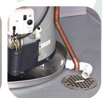
The Temperature and Pressure Relief Valve (T&P) discharge pipe should be terminated near a floor drain with an air gap of no more than 6 inches between the end of the discharge pipe and the drain. Some localities require terminating the T&P discharge pipe outside. In cold climates, we recommend using a floor drain. In all cases, follow local codes. Read the Instruction Manual for important details. Warning: Do not plug or cap the T&P discharge pipe.
