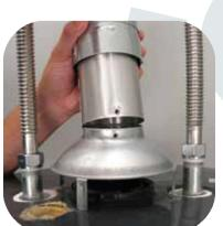
Be certain that the vent has cooled before handling. Disconnect the vent pipe from the draft hood. Gas water heaters must have free access to adequate combustion air and must be properly vented. The Installation Instructions explain these requirements, and they must be followed for safe operation.
