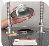
Connect the vent pipe to the water heater's draft hood. Use sheet metal screws. Don't reuse the old draft hood—always use the new draft hood supplied with your new water heater. See the Installation Instructions for important safety information about venting and construction details.
