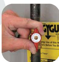
Turn the gas supply valve ON. Brush soap solution on all gas line connections and look for bubbles. Use plenty of soap solution. Gas is under low pressure, and it may take some time for bubbles to appear.
