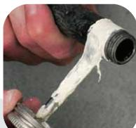
Install the gas pipe using pipe joint compound (or Teflon® tape) approved for fuel gas on all threaded connections. Keep the pipe joint compound from getting inside the gas line or gas control valve. If you are using a flexible gas line connector, follow the instructions that came with the flexible connector (most don't need pipe joint compound). Reconnect the gas line union.
