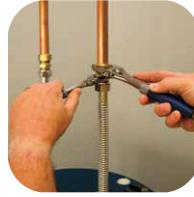
Install the hot and cold water lines. The water heater inlet and outlet connections contain non-metallic parts. Don't solder pipe directly to these connections. Instead, solder threaded adapters to short pieces of pipe so that soldering is done a foot or so from the water heater connections. Open the cold water supply valve and fill the tank.
