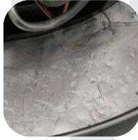
Gas water heaters produce condensation the first time they are started up. You may hear drips (or a sizzling sound as droplets hit the burner) or you may even see a small puddle. **Condensation is normal** and is not a leak. Condensation should go away when the water heater reaches its normal operating temperature. Check the water connections for leaks. Most actual leaks occur at the inlet or outlet water connections—not a tank leak.
