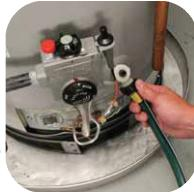
Connect a garden hose to the drain valve. Place the other end of the hose in a drain or outside (you could also use buckets). Shut off the cold water supply to the water heater and open a hot water faucet and the drain valve. While the water heater is draining, read the Installation Instructions that came with your water heater.
