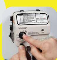
Follow the lighting instructions on the water heater's label. Turn the control knob to Pilot and press the knob in. While holding the knob in, click the igniter button about once a second until the Status Light begins to blink (this may take up to 90 seconds).
