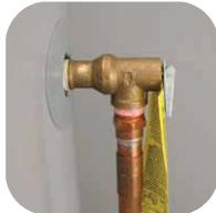
The Temperature and Pressure Relief Valve (T&P) is an important safety device. It opens to relieve pressure if the water temperature or pressure is too high. Use the new one that came with your new water heater. Don't reuse the old T&P valve.
