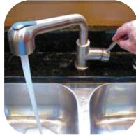
Open a nearby hot water faucet. At first, you'll just get air from the faucet, then sputtering, and finally, a full flow. Then, let the "hot" water run full stream for three minutes to ensure the tank is completely full. The tank must be completely full before lighting the pilot.
