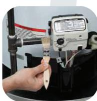
If you see any bubbles, turn the gas off, correct the leak and retest.
