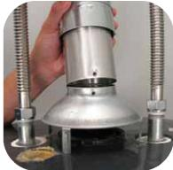
Disconnect the vent pipe from the draft hood. Gas water heaters must have free access to adequate combustion air and must be properly vented. The Installation Instructions explain these requirements, and they must be followed for safe operation.
