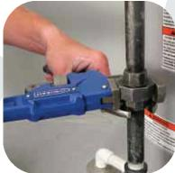
Disconnect the gas line at the union (you'll need two wrenches for that). Remove the gas pipe from the old water heater—you may be able to reuse it. Save the union, too. Next, remove the water lines and the old water heater. Inspect the old vent pipes for corrosion, obstructions, leaks or other damage, and repair or replace if necessary. Install the new water heater in a metal drain pan.
