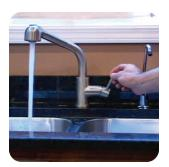
*Remove trapped air from the other side of the bladder by turning a hot water faucet on until a steady stream flows.* An Expansion Tank can help prevent damage to pipes, appliances, and the water heater itself.
