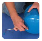
Check the air pressure in the Expansion Tank using a tire gauge.
