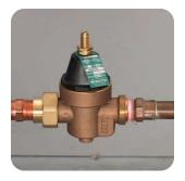
If the water pressure is greater than 80 PSI, install a Pressure Reducing Valve. The recommended water pressure is between 50 and 60 PSI.
