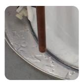
Drips from the Temperature and Pressure Relief Valve are usually caused by (1) water pressure too high, (2) lack of Thermal Expansion Tank.
