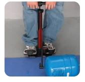
Adjust the air pressure to equal the maximum water pressure in the home. Use a hand pump - **NOT** an air compressor - or you may rupture the bladder.
